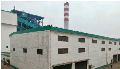
Solid Waste Incinerator of Chongqing Lee & Man 重慶理文固廢焚燒爐
